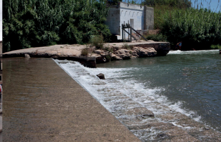
Tormos irrigation dam
